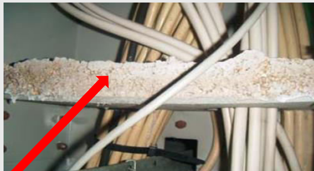
Insulating board with non-asbestos sprayed coating
