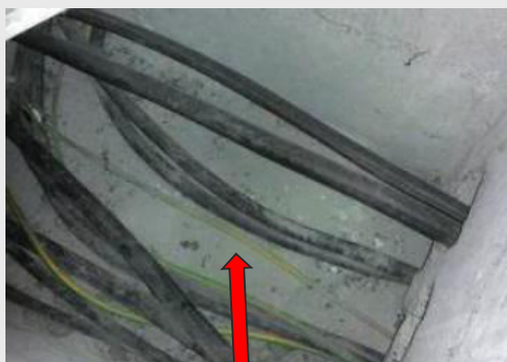
Cable run with dust/debris
