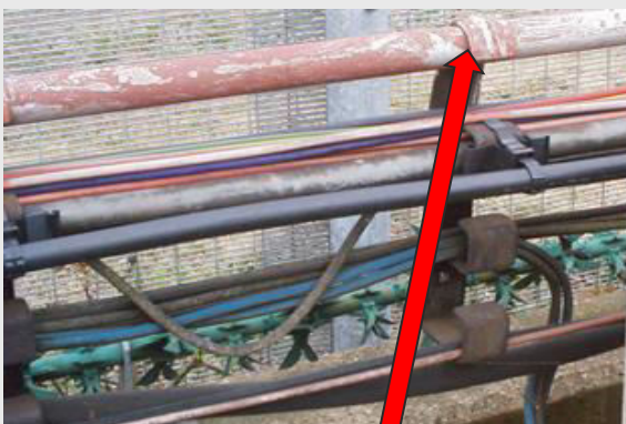
Packing to cable hangers
