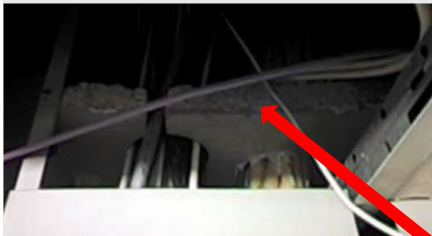
Insulating board with non-asbestos sprayed coating
